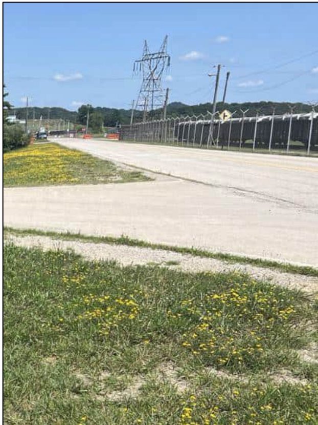
Representative photo of impervious surface
